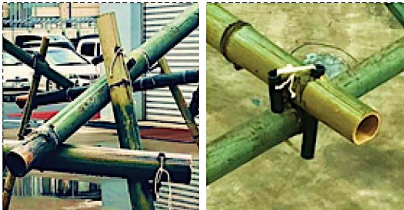
Figure 11: Joint using PVC pipes and ropes
