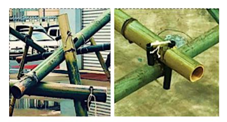
Figure 11: Joint using PVC pipes and ropes
